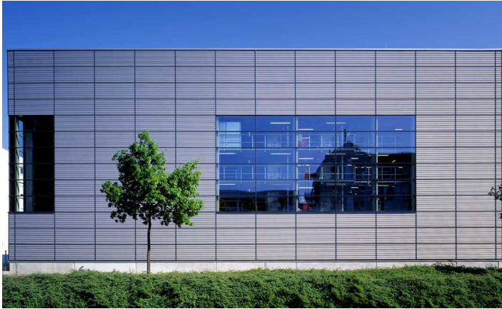
Detail Fassade Rotationshalle
